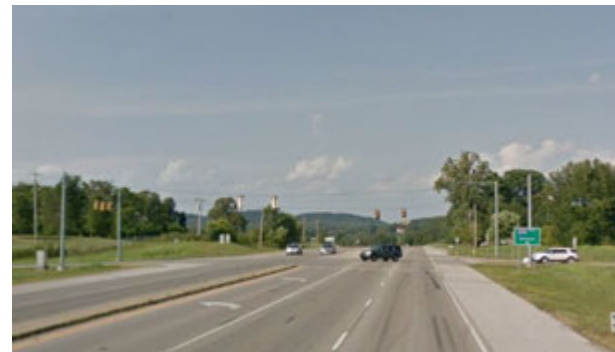
Columbia Pike (SR 6/US 31) Looking North at I-840 Westbound Ramp
