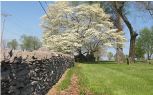
View of the existing rock wall along Columbia Pike.
