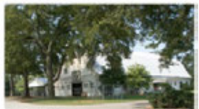
View of existing barn.
