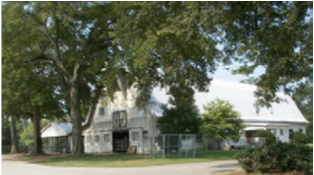
View of existing barn.
