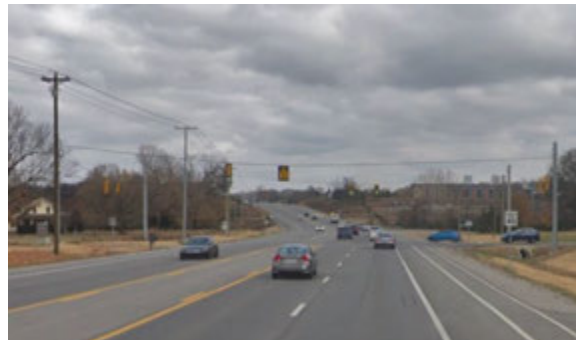
Columbia Pike (SR 6/US 31) Looking North at Critz Lane
