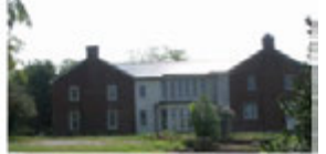
View of the preserved Roderick House.
