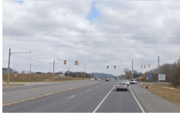
Columbia Pike (SR 6/US 31) Looking North at I-840 Eastbound Ramp
