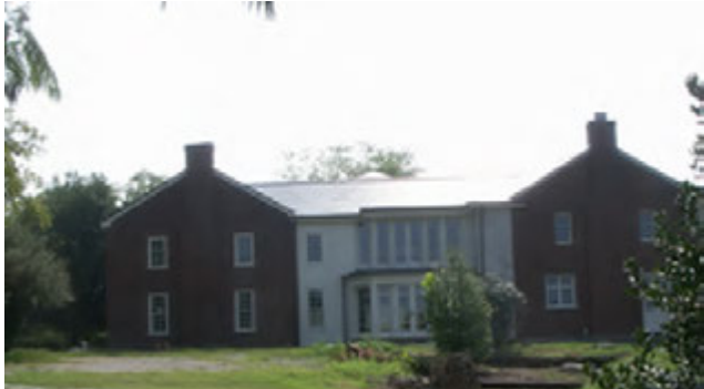
View of the preserved Roderick House.
