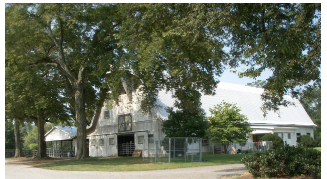
View of existing barn.
