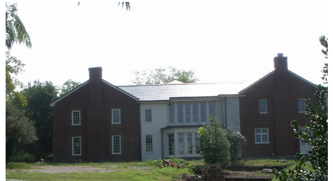
View of the preserved Roderick House.
