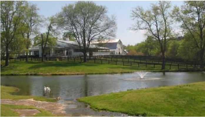
View of the existing structures overlooking the pond.
