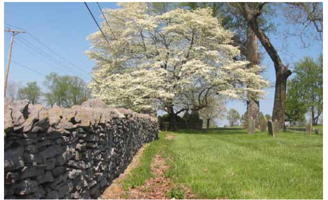
View of the existing rock wall along Columbia Pike.
