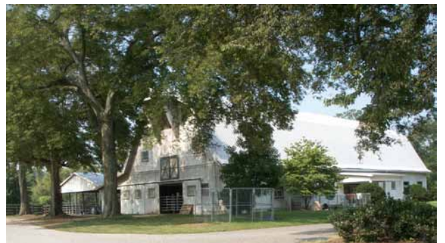
View of existing barn.
