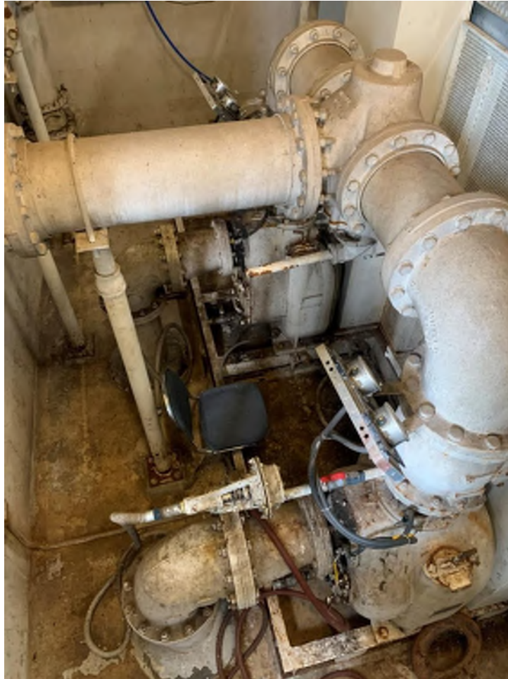
Figure 3.1 - Existing Influent Pump Station
