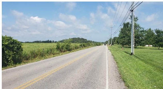
Thompson’s Station Road East looking east, south of the project site
