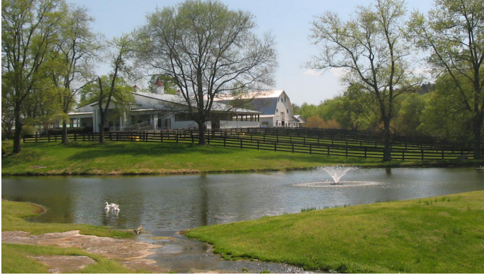
View of the existing structure overlooking the pond.
