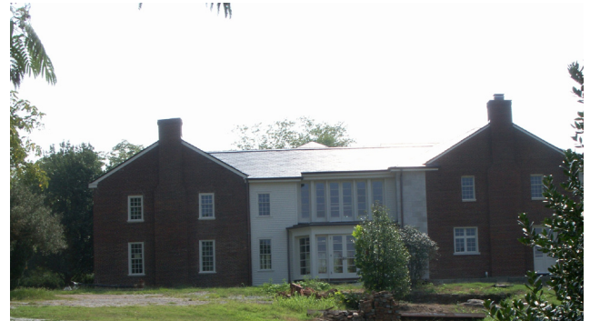
View of the preserved Roderick House.
