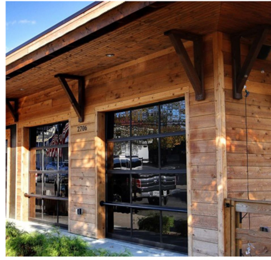
EXAMPLE OF ROLL-UP DOORS AT OUTDOOR PATIO
